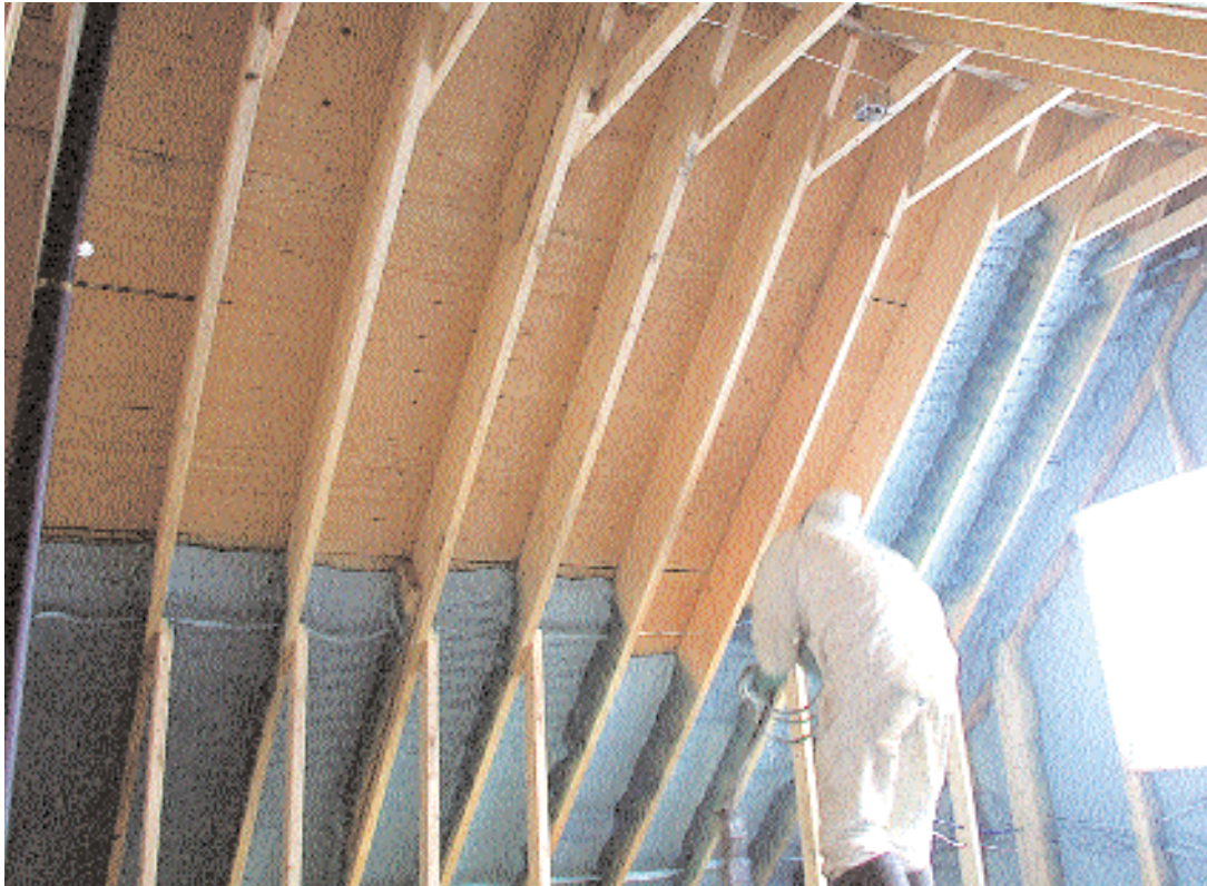
Photo courtesy of Great Northern Insulation
