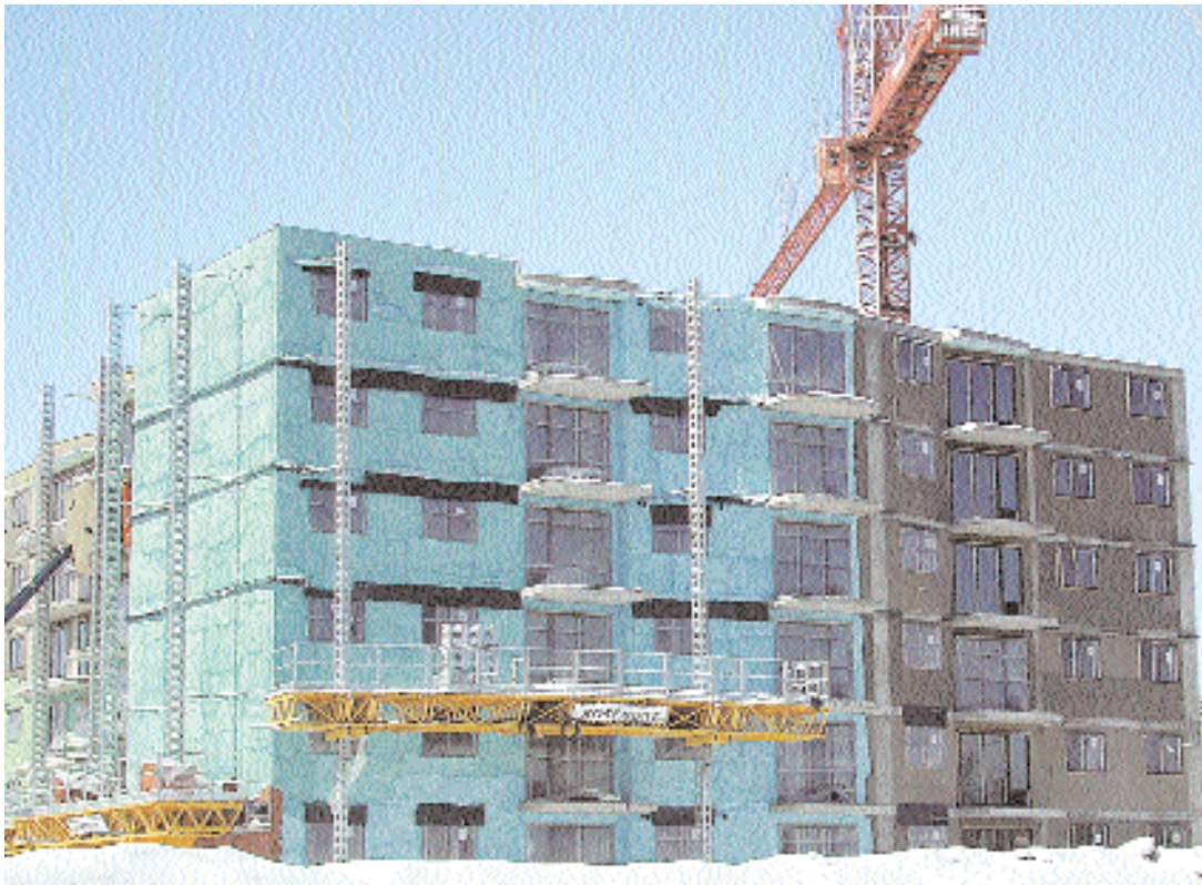
Photo courtesy of Great Northern Insulation
