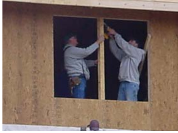
Figure 44. Structural support placed between two windows eliminates need for wood header.
