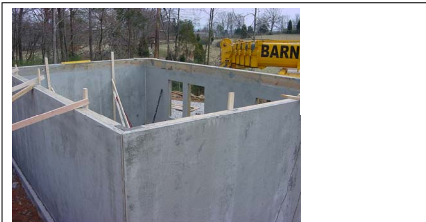
Figure 41. ZEH4 TMass foundation in place and ready for floor trusses.
