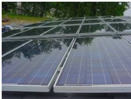
Figure 51. Modules are clamped to the rails.
