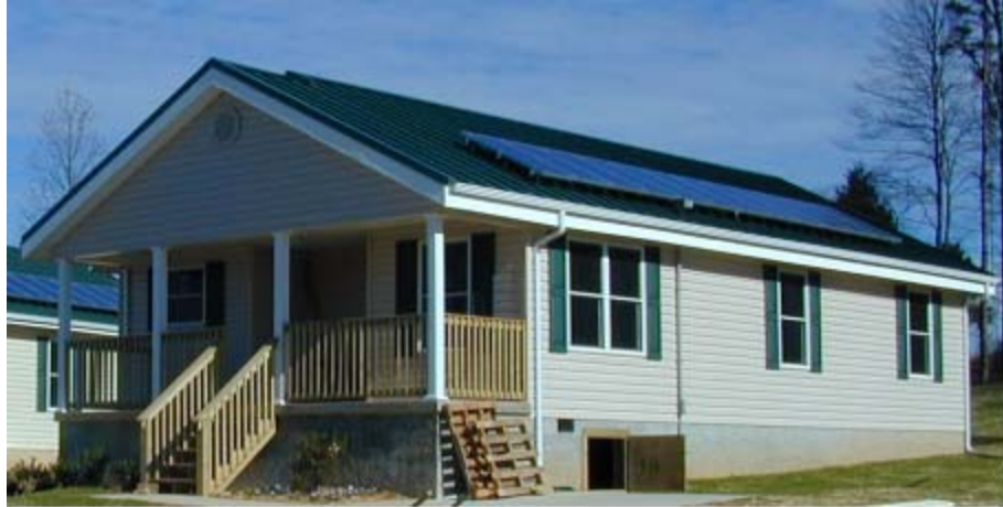
Figure 50. ZEH-3, with the twelve solar panels of the PV system on the roof.
