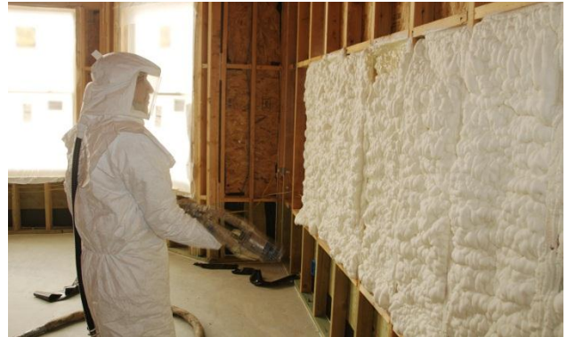
Figure 4 - Spray Foam in an Exterior Wall Cavity
